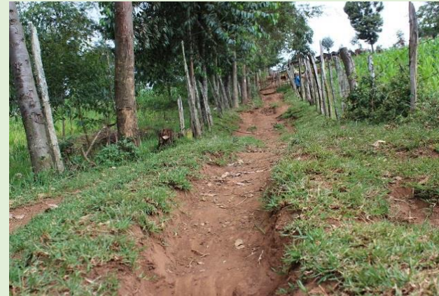
Figure 1. Path erosion channels sediment to the stream. Left untreated it can eventually form deep gullies.
